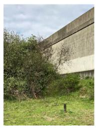
Temporary stability of the PFA embankment (up chainage of the existing wall) should be favorable when excavation into the existing embankment slope will be carried out to fit the lower layers of geogrid.
