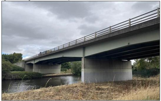
The alignment of the new deck shall provide 2m clearance from the existing bridge deck for future maintenance access. The new abutment is set out to avoid a clash with existing H piles. Sheet piles provide scour protection and additional sheet piles will extend this protection to the new piers. The new deck will be steel, hence compressive load on the new piles is modest and pile section is controlled by the lateral loads and moments.
