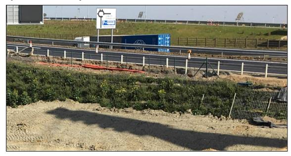
Tensar have provided advice and an application suggestion for TensarTech 'GreenSlope system' which is included in Appendix E. Initial geogrid lengths have been calculated to be approximately 75% of the height of the strengthen slope. This is considered an adequate level of design to inform the temporary works assessment of short-term excavations into the existing A46 embankment slopes and in turn confirm the location of the new toe of batters.
